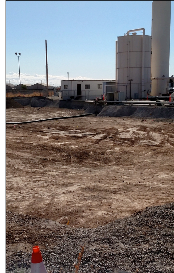
PRL020 – Completed soil excavation of area under northeast corner of the GWTP. Completed final status surveys. Preparing post remediation data package.
