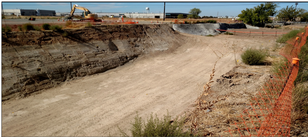
PRL020 – Completed soil excavation of area under northeast corner of the GWTP. Completed final status surveys. Preparing post remediation data package.
